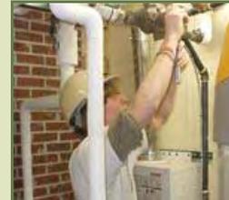
Tulsa Job Corps student, Jonathon Falgout, installs the valve on the new energy-efficient hot water heater.
